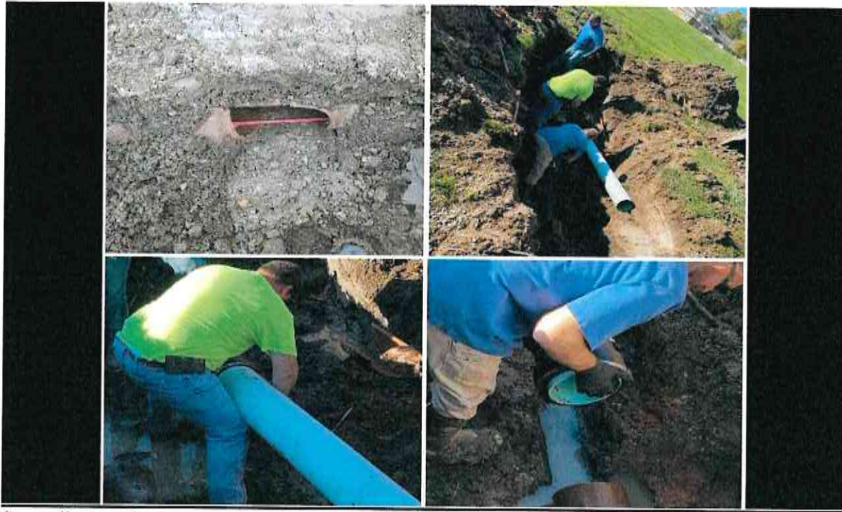
Sewer line repairs on Henry Clay
