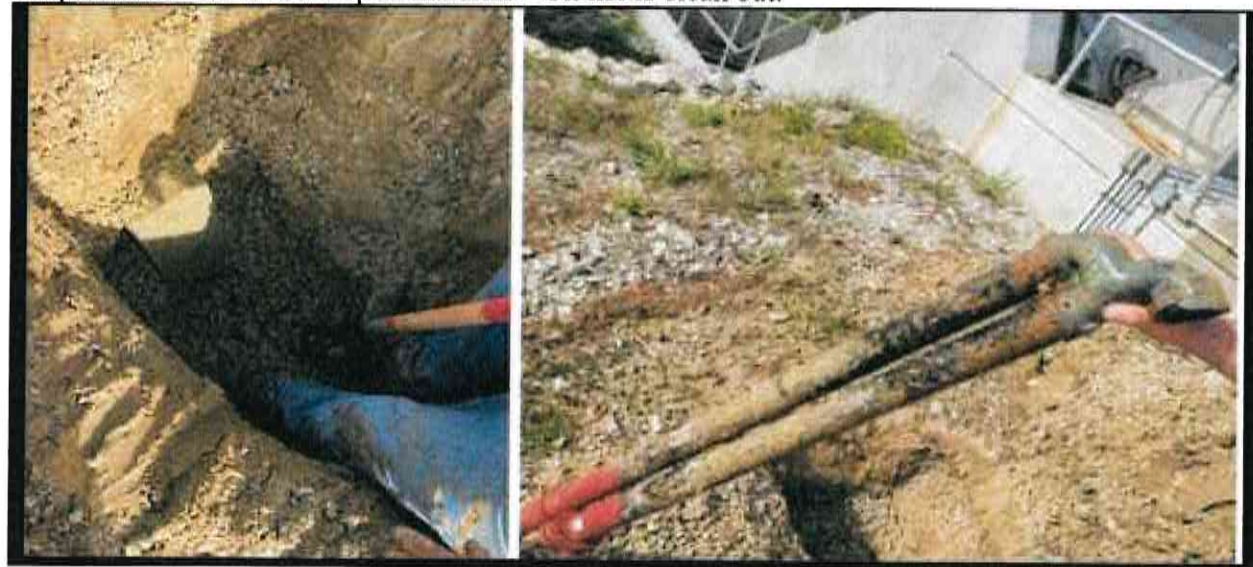
Waterline repairs at WWTP
